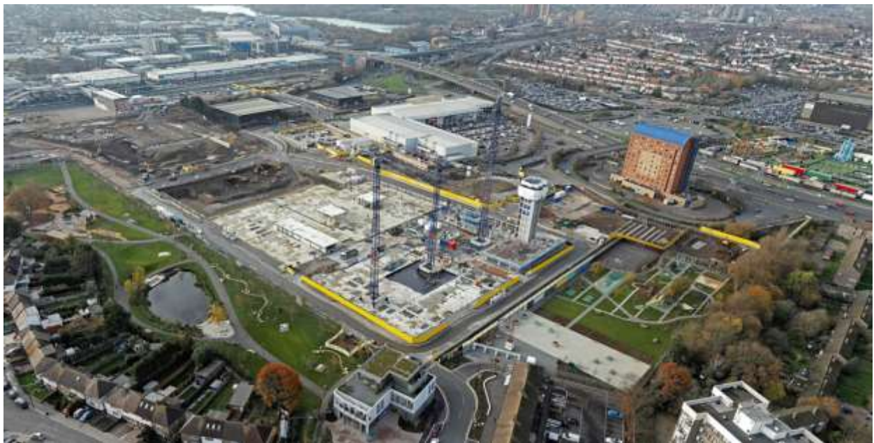
First tower cranes constructed and core of plot 12 now visible above ground (December 22)
