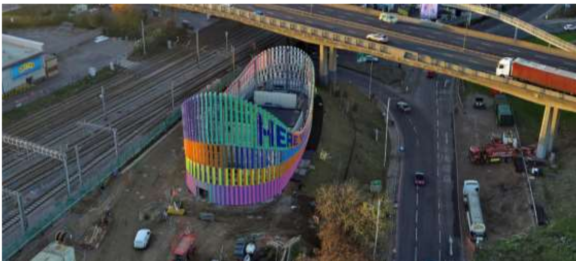
Brent Cross Town primary substation wrap complete
